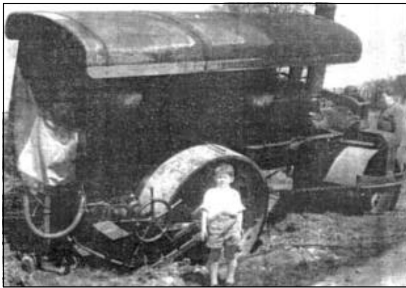
Ditched steam roller
